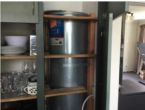
11. 180L mains pressure HWC manufactured 2011
