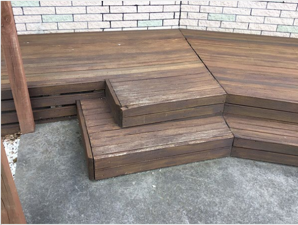
25. Deck due for recoating
