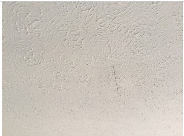
22. Cosmetic ceiling crack in bedroom 1
