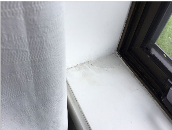
21. An example of unfinished reveal repairs
