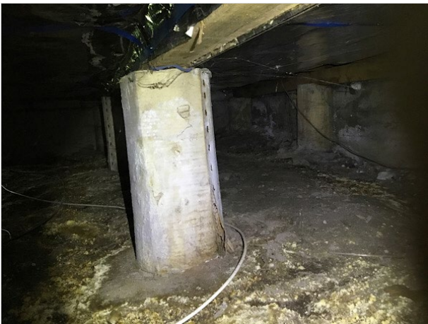
9. Typical pile and subfloor moisture barrier
