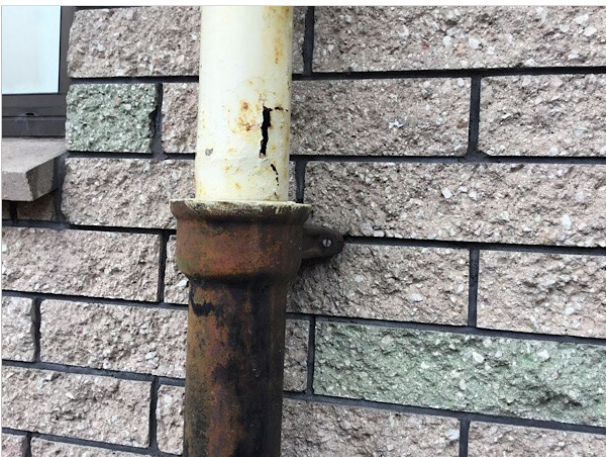
23. Sewer vent pipe corroded
